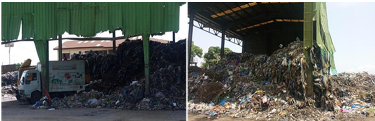
Plate 9.3: Left: Stockton Creek Transfer Station (truck dumping without using the ramp); Right: Fiamah Transfer station, with waste spilling out of the protected bay
