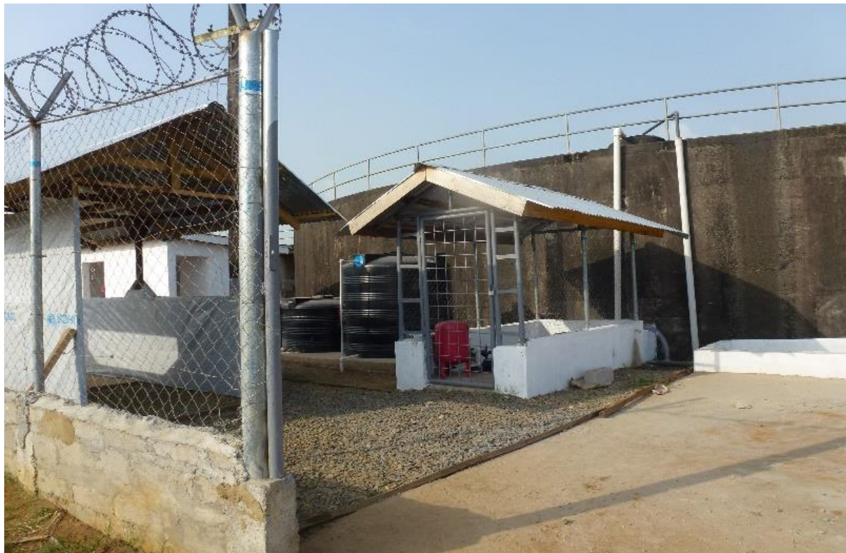
Plate 9.2: Disposal site at Liberia Water & Sewer Facility at Fiamah
