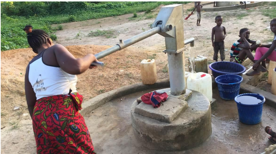
Plate 7.1: Hand pump creates access to groundwater (Greencons, 2019) 18
