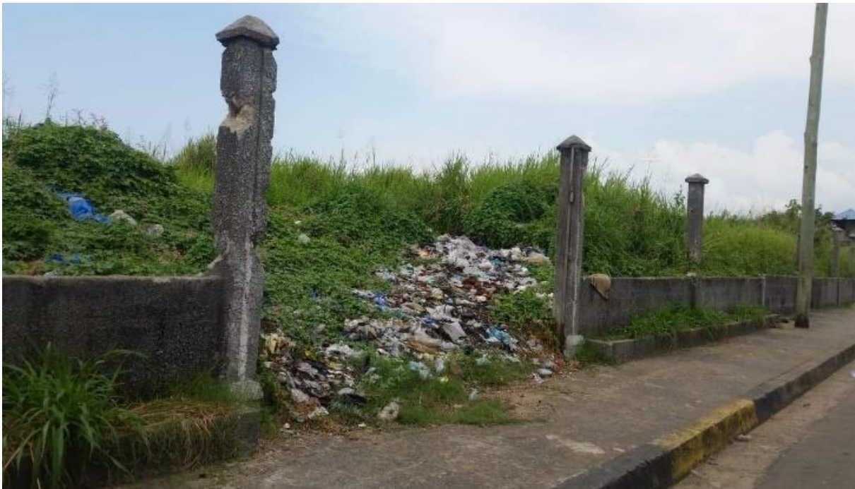
Plate 9.6: Waste dumped in Palm Grooves Cemetery (source: Greencons)
